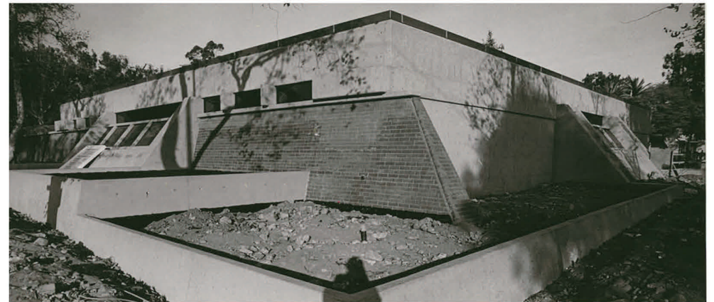
Construction and completion of the new library building, 1974-75.
